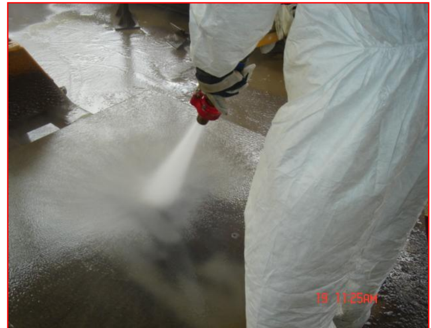
The Wet Abrasive Blast System with controlled pressure, water and media capabilities
